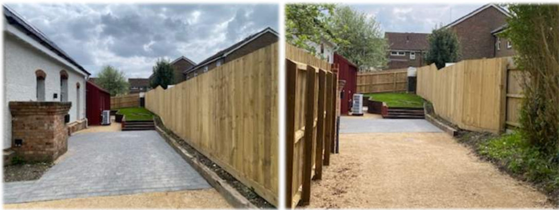
Figure 1.5 (above) Views of the rear (east) elevation.
