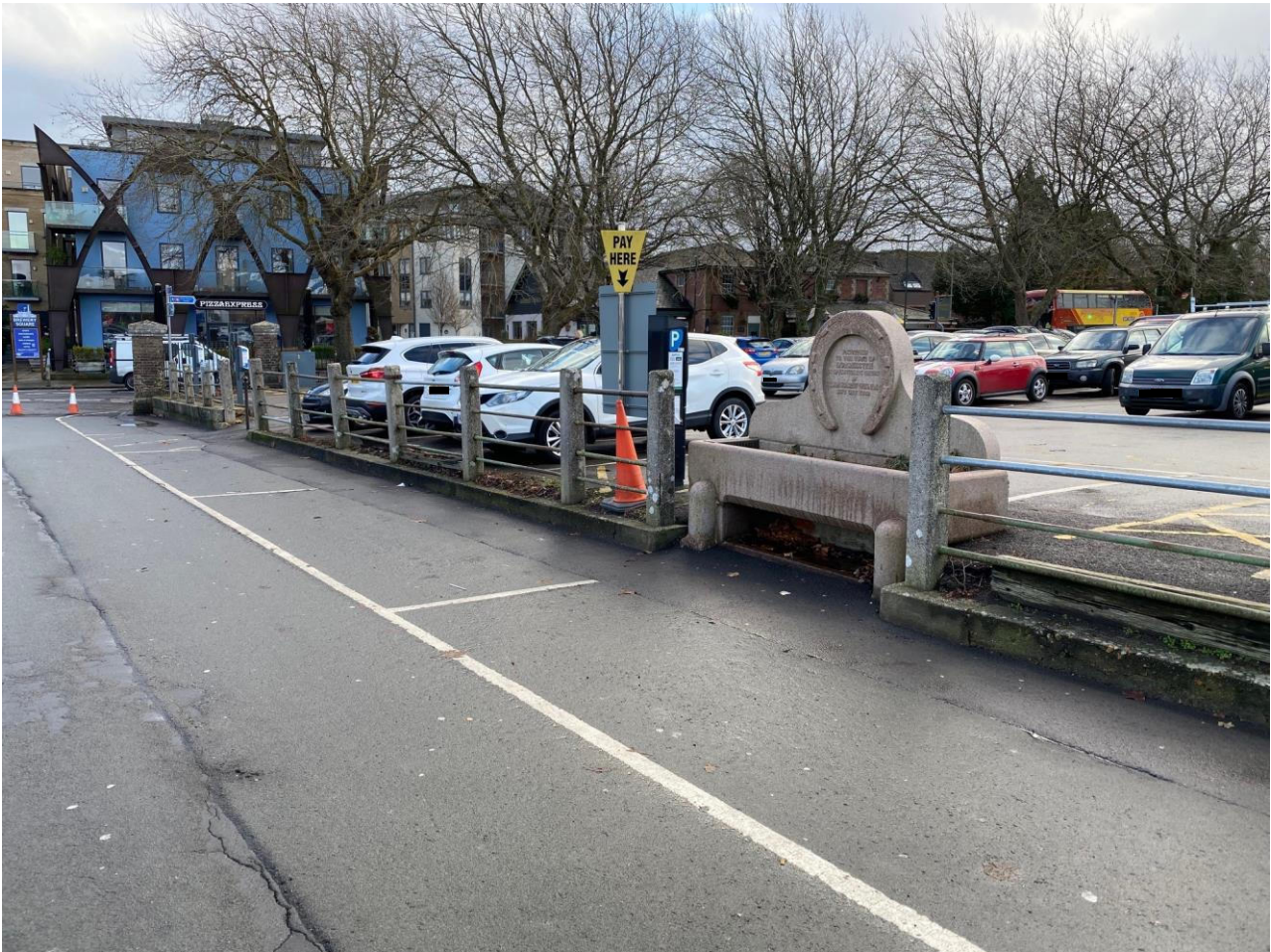
Figure 7. The granite horse trough located on the south side of Fairfield Road
